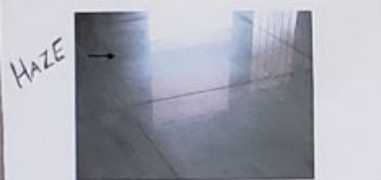
Photo No. 2. Note the shadow line on the left becomes hazy about half way down. This localized loss of reflectivity is being called optical hazing in the tile industry.
